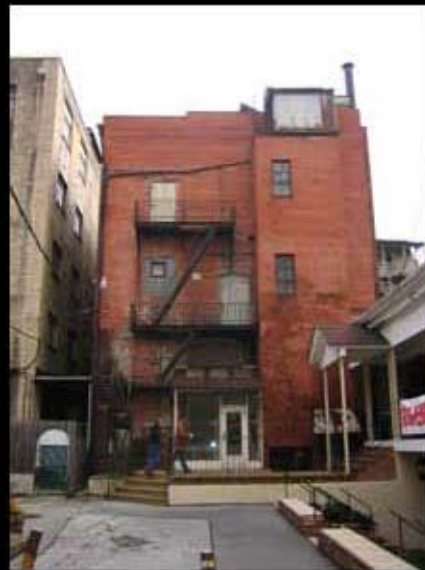
Rear facade c. 1950s
