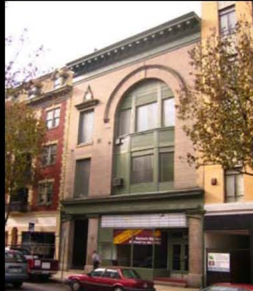
Front facade before
